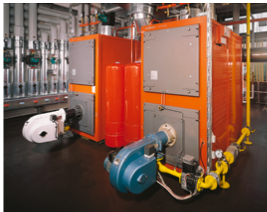
Gas inlet pressure monitoring on high-performance boilers
