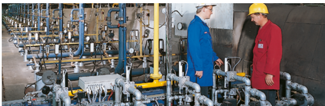
Gas train in a brickworks
