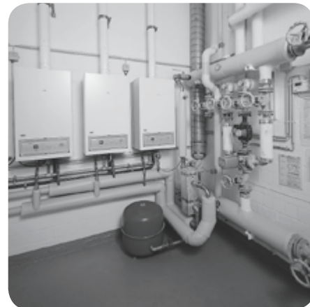
Heating boilers connected in cascade
